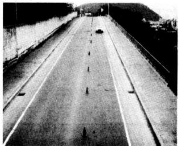
Figure 7. By May, snow has almost completely melted, and the road's lines are redefined.
